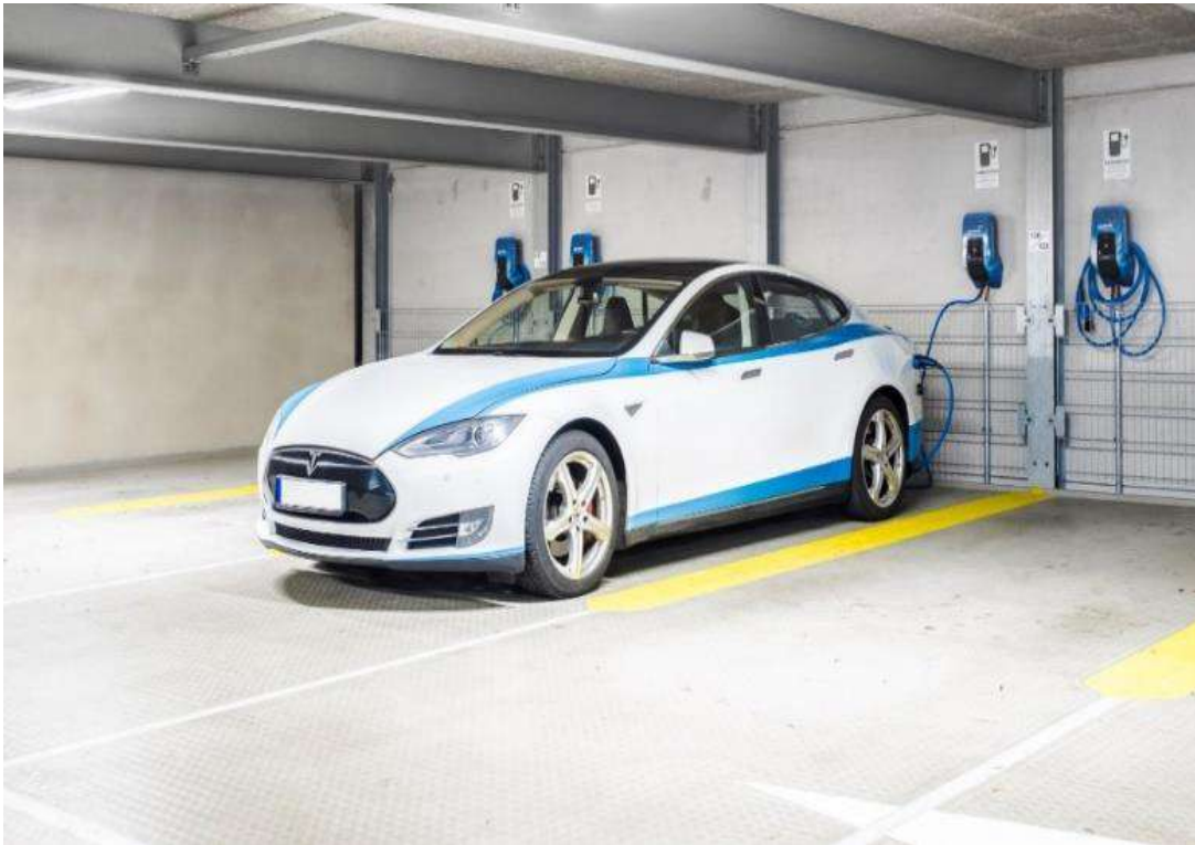
Parking garage Hamburg warehouse district
